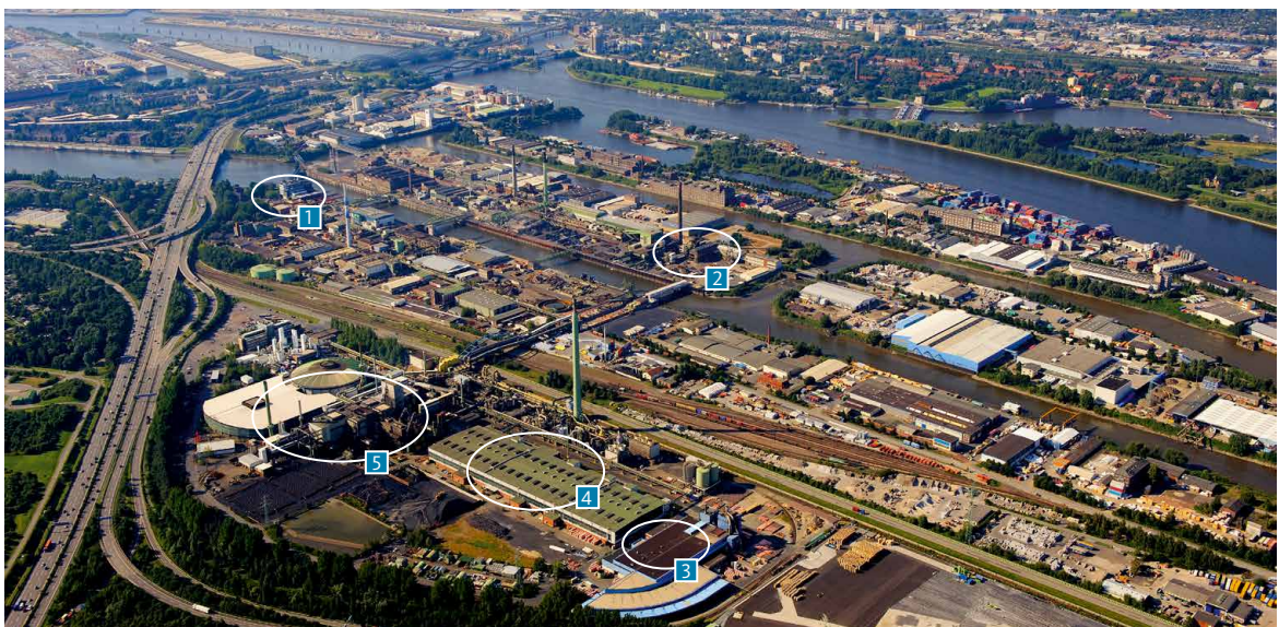
1 Continuous casting plant 2 Secondary copper smelter/precious metals 3 Rod plant 4 Tankhouse 5 Primary smelter (RWO)
