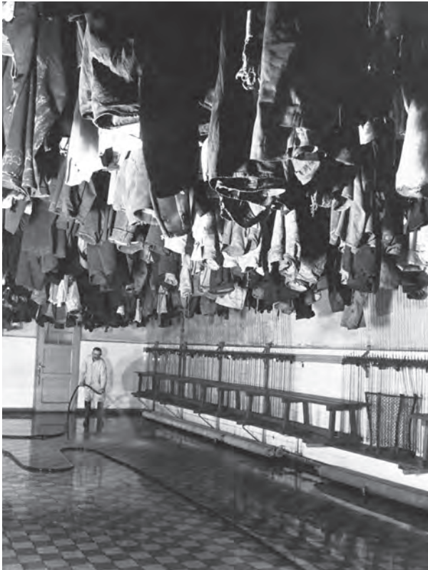
In 1927, NA built a washhouse specifically for its employees to help improve standards of hygiene and thus workers' health. After every change of shifts it was tidied up and cleaned.
