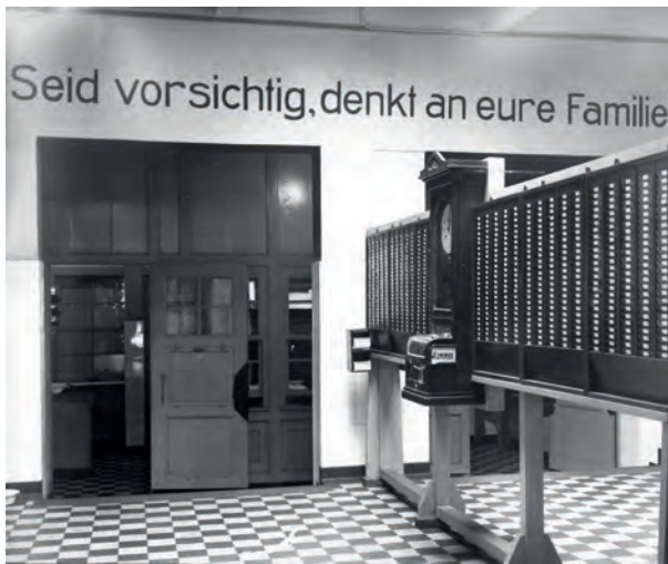
The company has always called on people's individual responsibility and appealed to them to be careful in their work, as can be seen here in large letters on the wall of the social services building around 1930 ("Be careful, think of your family!"). The time clock for recording working hours can be seen in the foreground.
