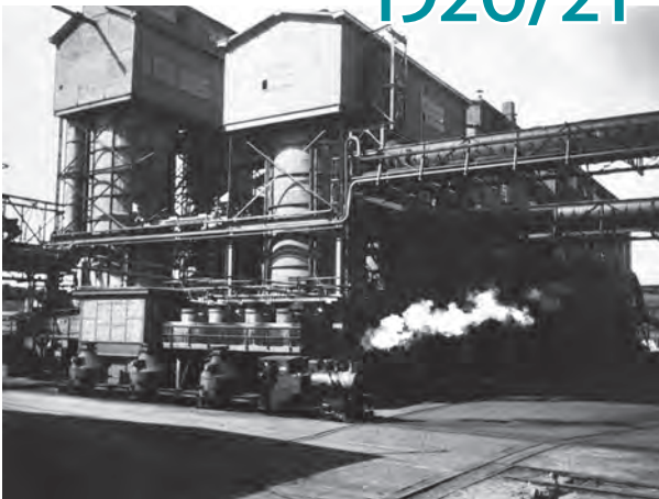
First utilization of coolers and fabric filters
