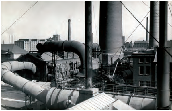
Beginning in the 1930s, flue dust systems not only kept the air cleaner but also held back sizeable amounts of valuable particulate raw materials which could thus be recovered.
