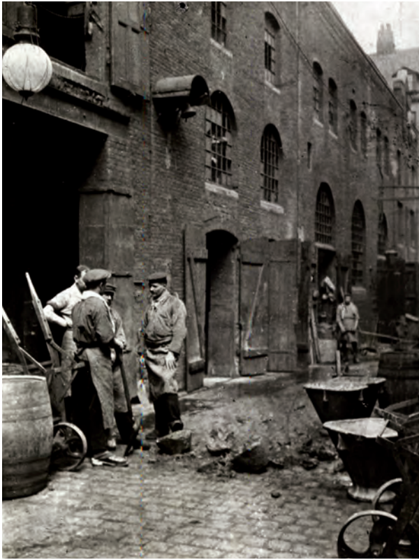
The courtyard of the plant at Elbstrasse with the gateway from Elbstrasse. On the left, the shaft furnace building with slag ladles and workers in the front.
