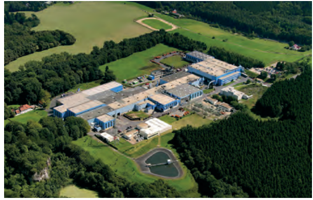
Stolberg is also home to Schwermetall Halbzeugwerk GmbH & Co. KG with a 300-strong workforce. They produce about 216,000 t of pre-rolled strip annually. The market leader for copper and brass pre-rolled strip is a 50 % subsidiary of Aurubis AG.
