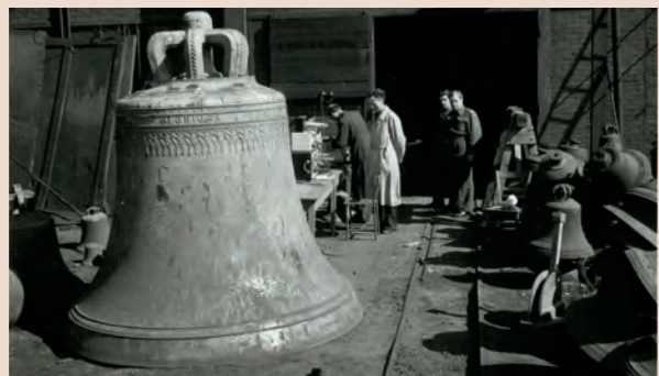
At the front, the “Gloriosa”, the largest bell from the Kaiserdom St. Bartholomäus in Frankfurt/Main, which survived the war at the Hamburg “bell graveyard”. The photo shows the “ring test” carried out by acoustics engineer Dr. Thienhaus in front of the southern wall of the reverberatory furnace building on the works premises.
