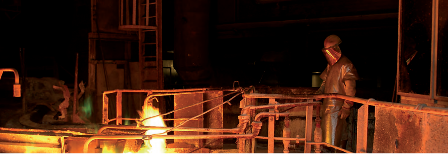
Anode casting wheel at the primary smelter (RWO). The newly built primary smelter started operation on March 9, 1972 and has stood the test of time.
