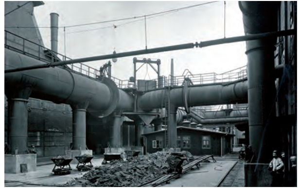
Flue gas pipes at the Hamburg plant in the 1920s.
