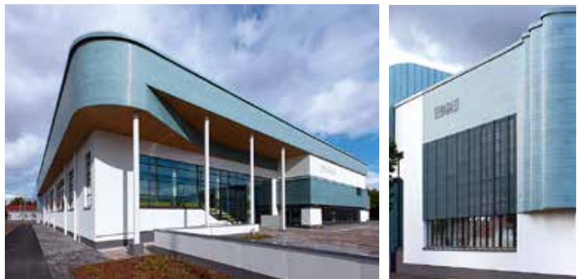
The award-winning copper solar façade system at the swimming pool in Pori
